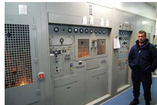
LORAN Transmitter Spaces
