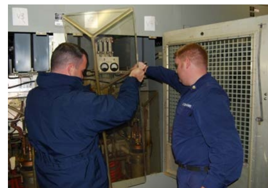
Insertion of acrylic-lead radiation shield
