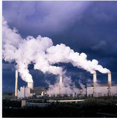
Routine Operation of Coal-fired power plants
