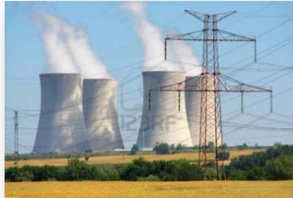
Routine Operation of Nuclear power plants
