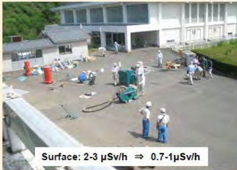
Decontamination of paved area by shot blasting
