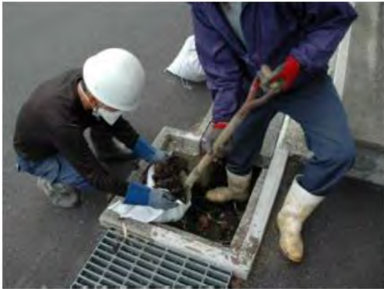
Removal of sediment in side ditches, etc.
