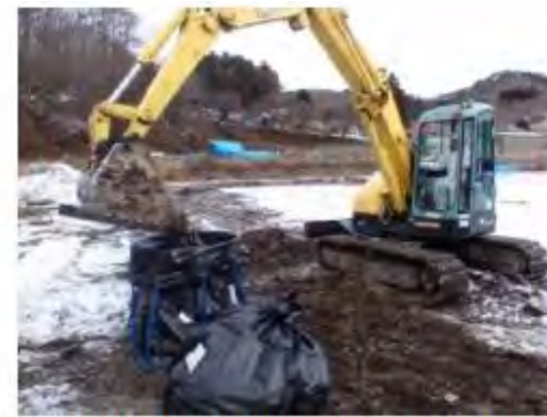
Topsoil stripping (mechanical digger)
