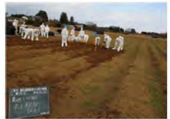
Manual topsoil stripping
