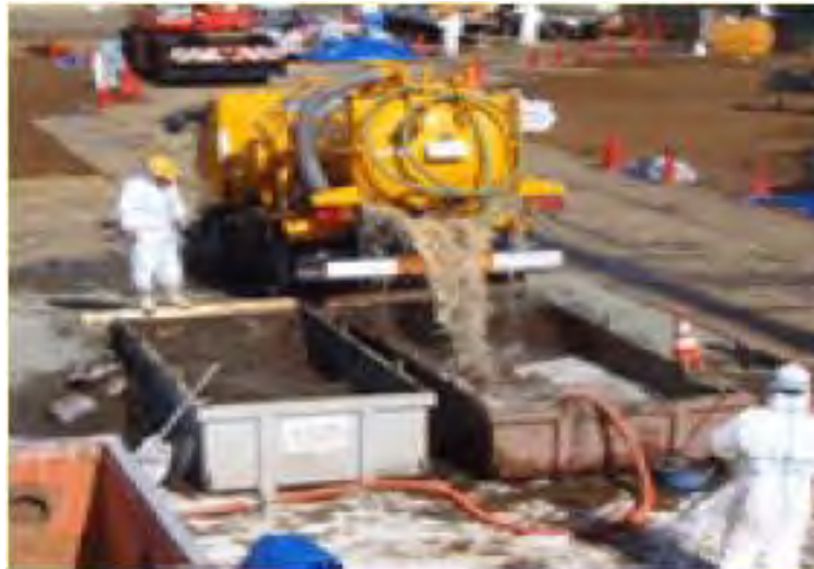
Transfer of water from vacuum tanker to treatment tank
