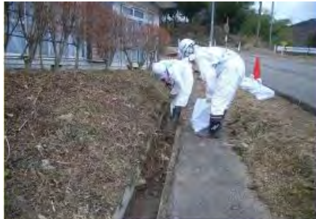
Removal of debris from drains
