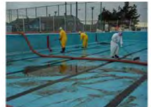
Figure 2-26: Decontamination of swimming pools
