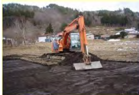
Stripping topsoil
