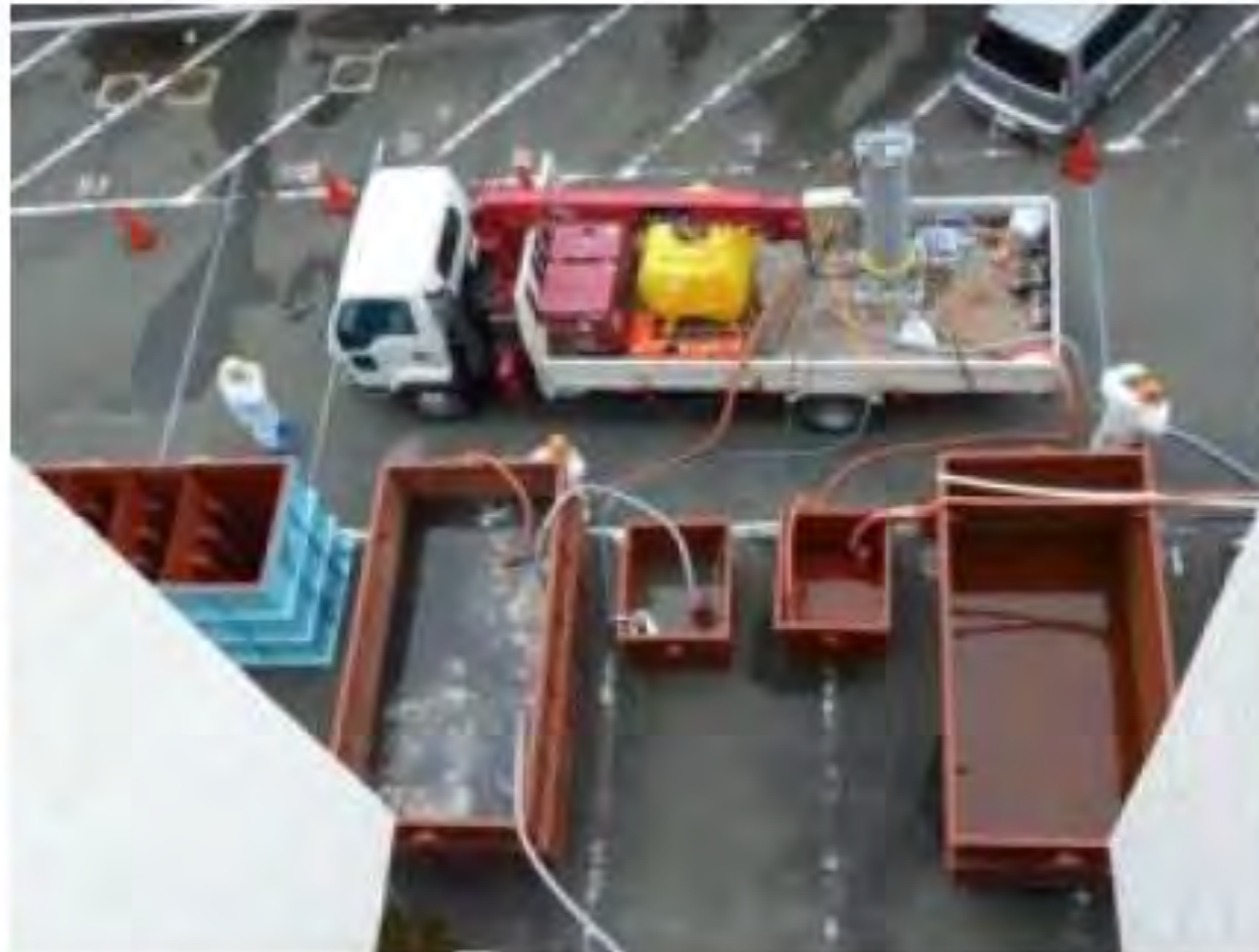
Figure 2-27: Decontamination of liquid waste: flow chart and equipment
