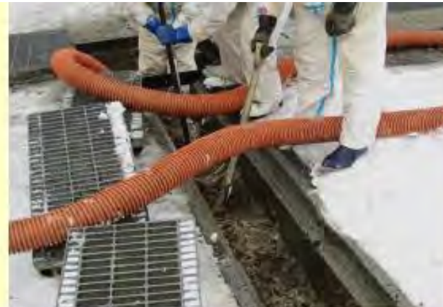
Removal of debris from drains
