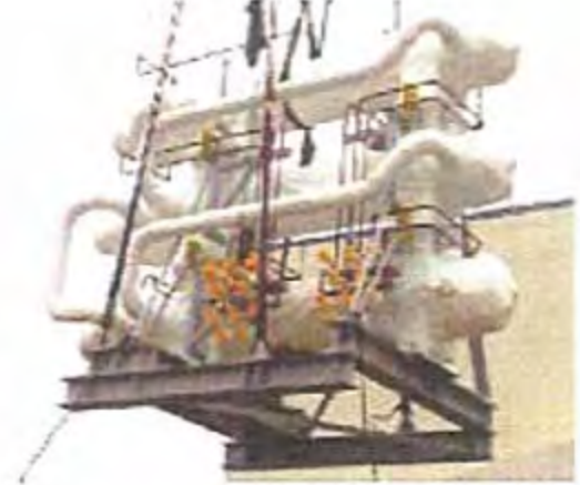
CUW Heat Exchanger Module
