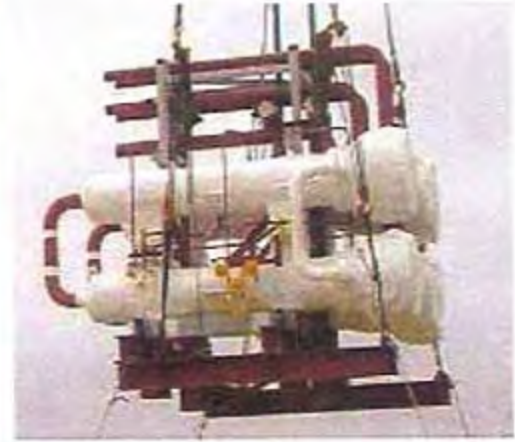
CUW Reheat Exchanger Module
