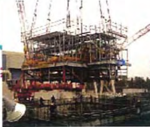
Piping Unit in T-G Pedestal Module
